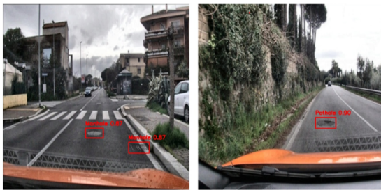
Fig. 4. Road Infrastructure and Hazard Detection using YOLOv11.
