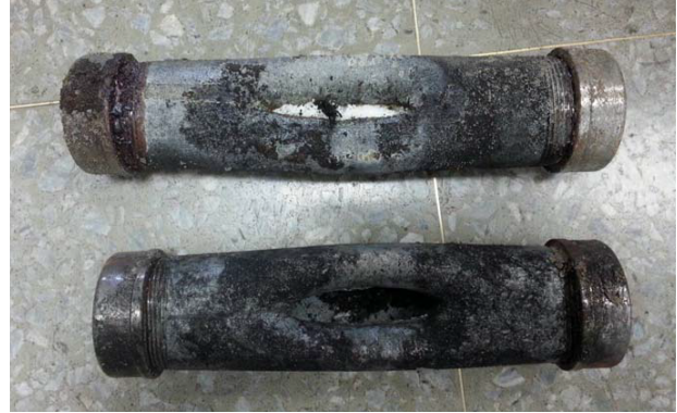
Fig. 16. The steel pipe ruptured by water jet impact (pipe thickness of 0.38cm).
