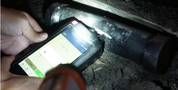
Fig. 14. Detect filled material by Raman Spectrometer.
